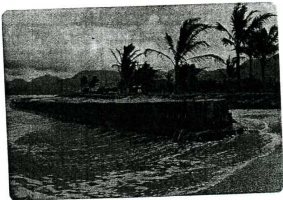
Figure 2-609. Seaward face of structure, Kualoa, Hawaii, 19 June 1978.
