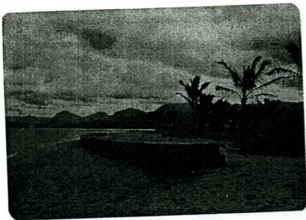
Figure 2-610. Sand accumulation on seaward face of structure, Kualoa, Hawaii, 4 January 1979.
