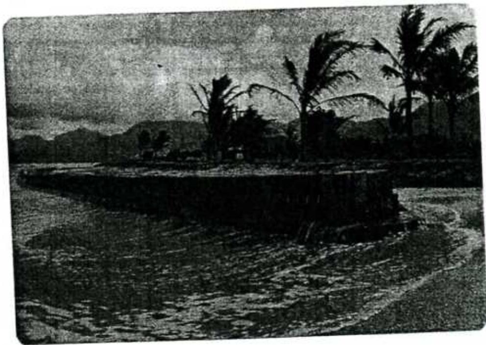
Figure 2-609. Seaward face of structure, Kualoa, Hawaii, 19 June 1978.
