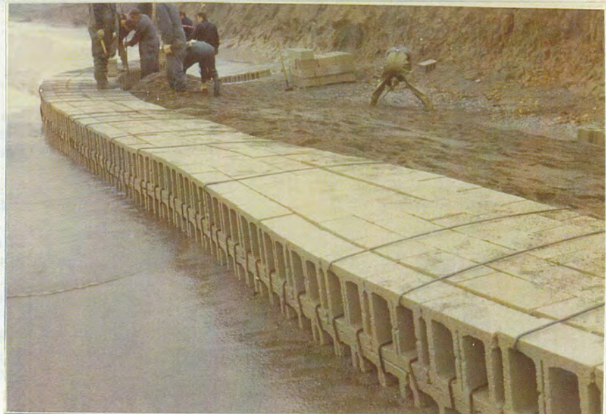
8th Day of Construction
