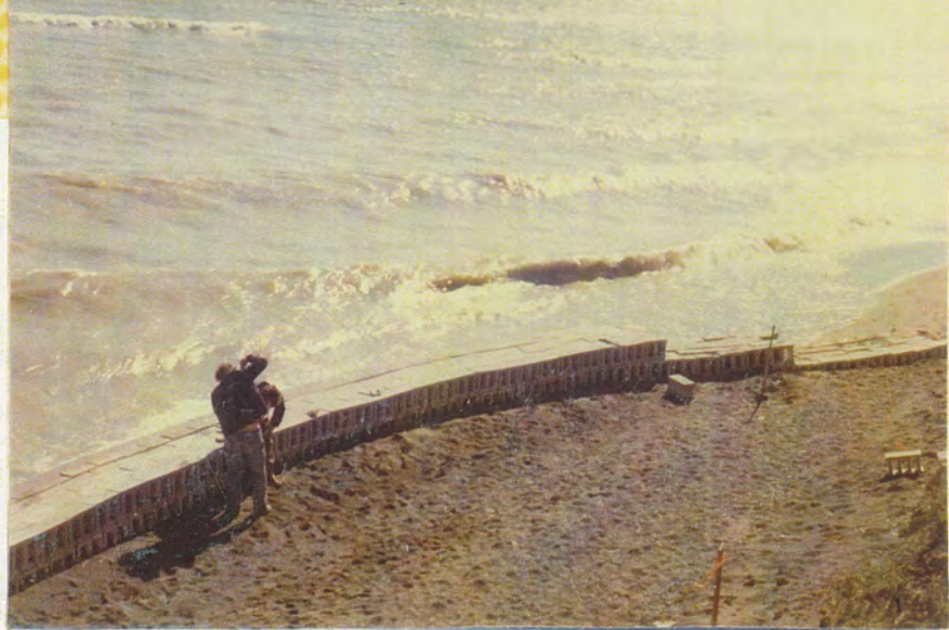
2nd Day of Construction
