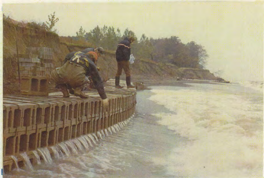
2nd Day of Construction
