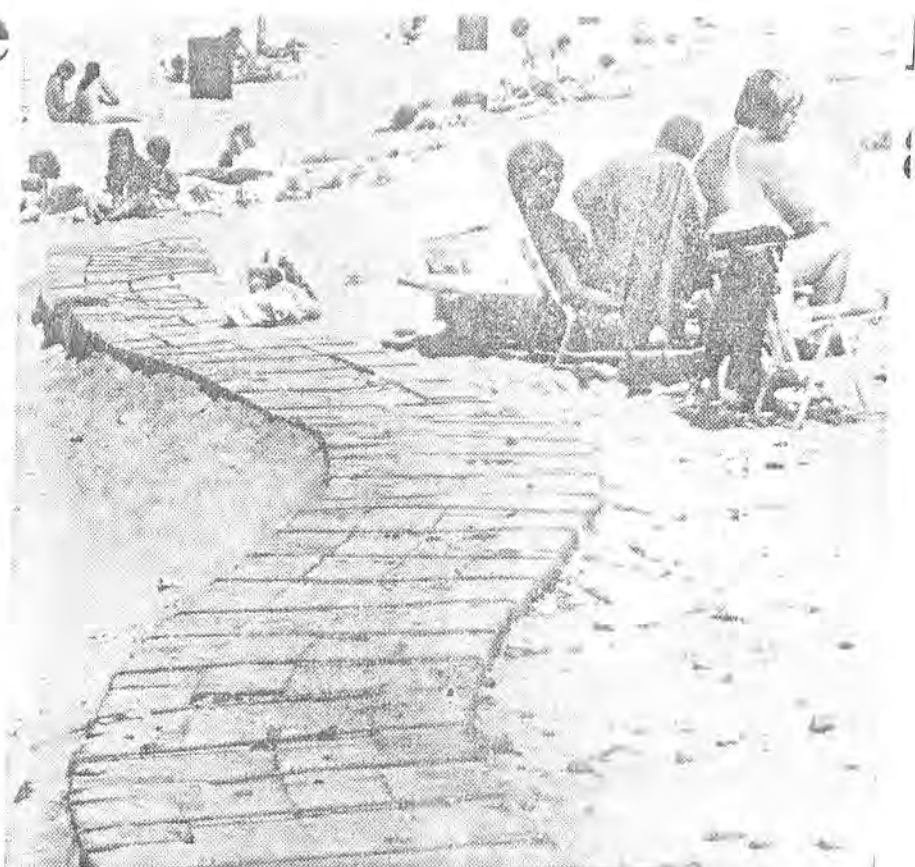
Cinder block breakwater prevents erosion at Duxbury Beach. STAFF PHOTO BY KEVIN COLE
