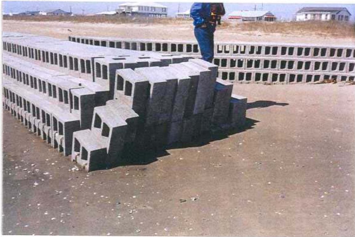
Figure 7. Settlement along the east end of the structure.
