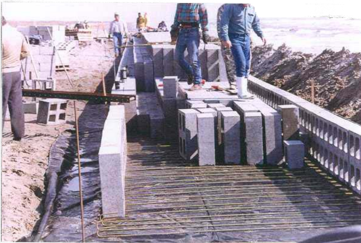
Figure 2. Parallel rows of concrete blocks as described in patent.
