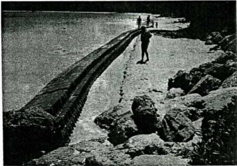
Figure 2-620. Seaward settlement of Sandgrabber, Bellows Beach, Hawaii, 5 September 1979.
