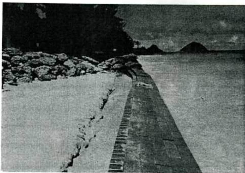
Figure 2-628. Scour trench along north end of structure, Bellows Beach, Hawaii, 5 September 1979.
