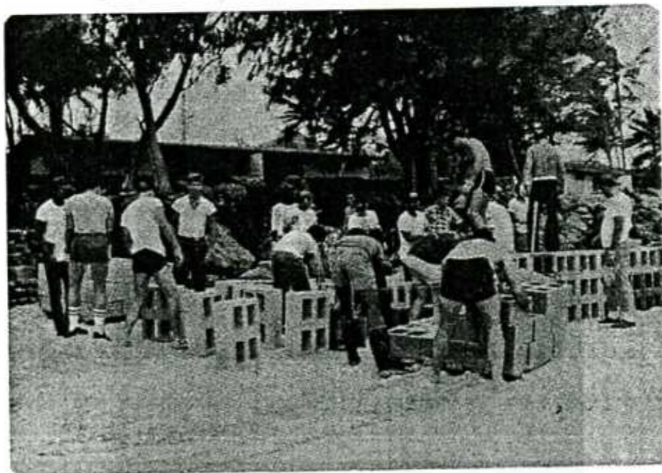
Figure 2-617. Placing blocks by hand, Bellows Beach, Hawaii, 8 February 1979.
