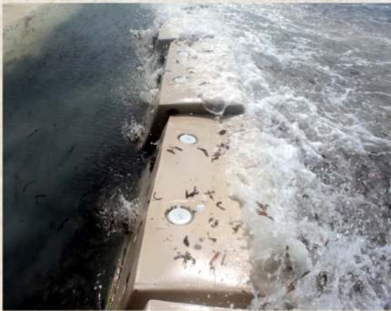
Wave Energy being dissipated as waves crash against Sandsaver™ modules. (Indian Ocean, Kenya)
